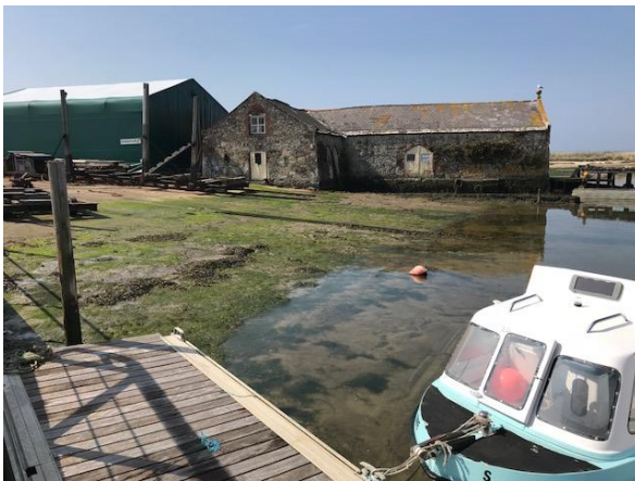
2: The Grade 2 Listed Yarmouth Sand House in the Harold Hayles Yard (David)
